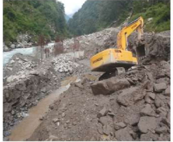
Excavation gravel trap
