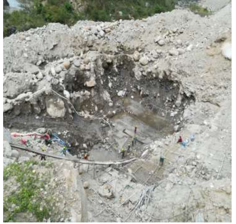
Power House Excavation गरिँदै
