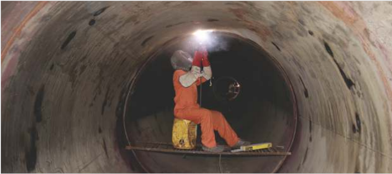
Welding of Penstock Pipe
