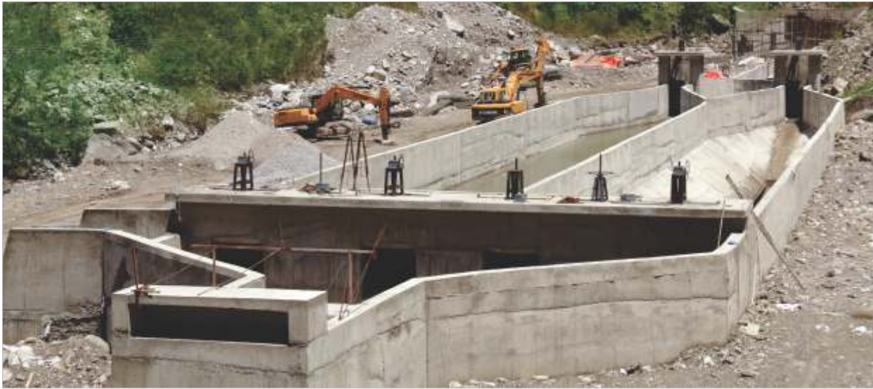
Forebay & Desander Basin
