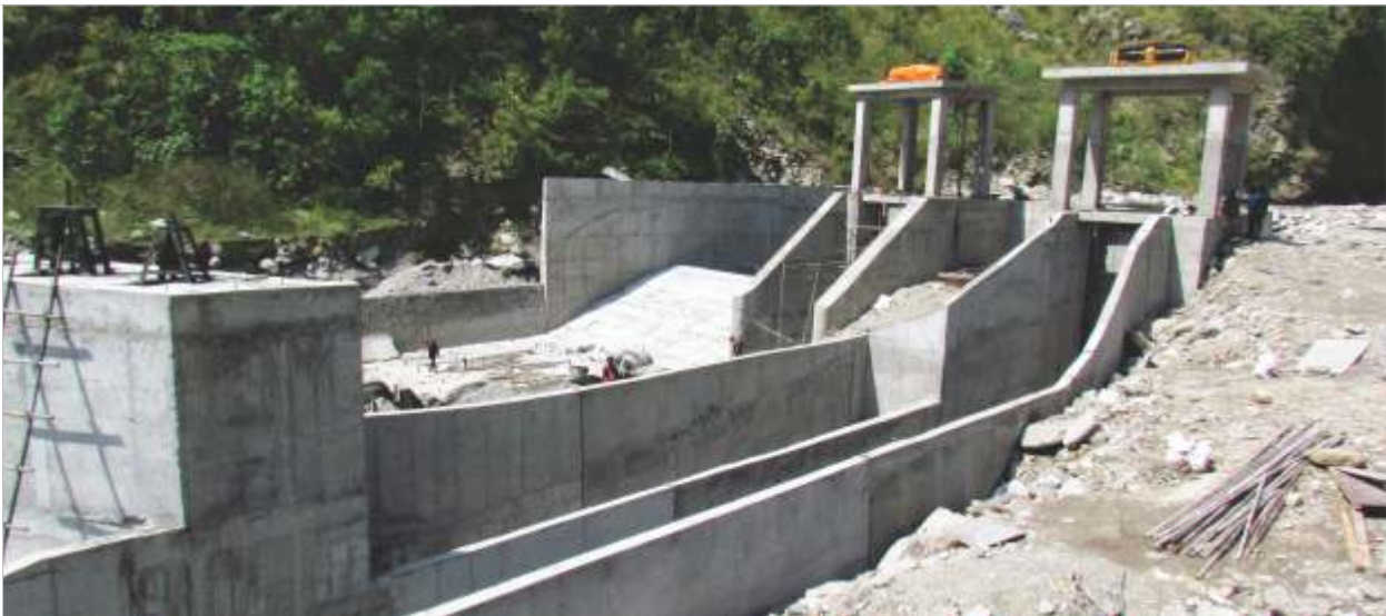
Installation of Inlet Gate & Hoisting System
