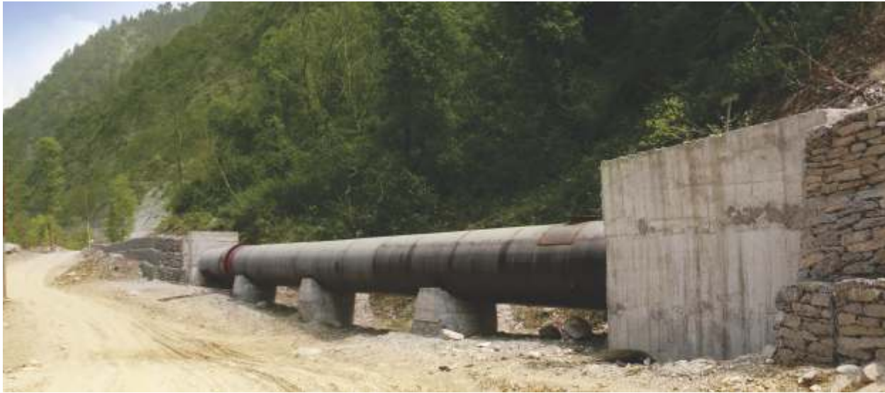
Anchor Block and Penstock Pipe
