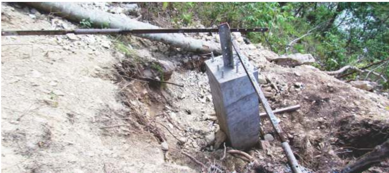
Concreting of Transmission Line Tower Foundation
