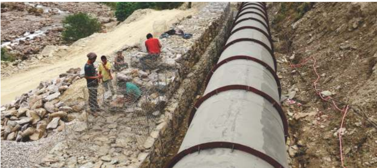
Gabion Protection Works for Penstock Pipe
