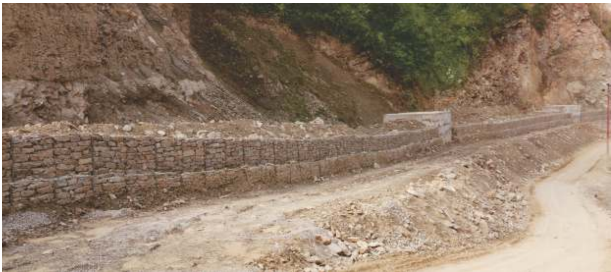
Protection of Penstock Pipe by Gabion Wall & Back Filling
