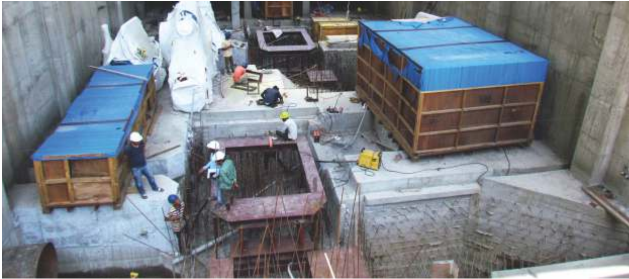
Installation of Electro Mechanical Equipment
