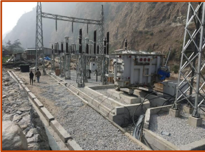
Power House Switch yard को कार्य प्रगति ।
