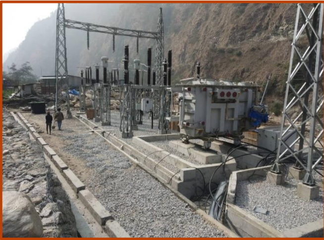
Power House Switch yard को कार्य प्रगति ।
