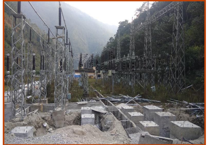
Singati Substation मा Bus Bar को foundation
